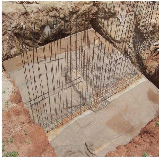
Figure 6 Showing the Foundation with partial Shuttering
