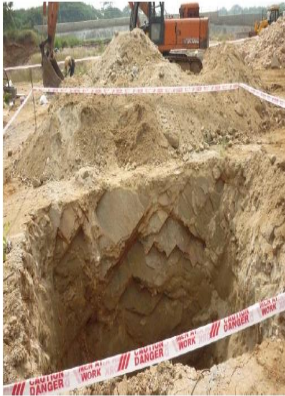
Figure 2 showing the Foundation pit showing soft rock at Site
