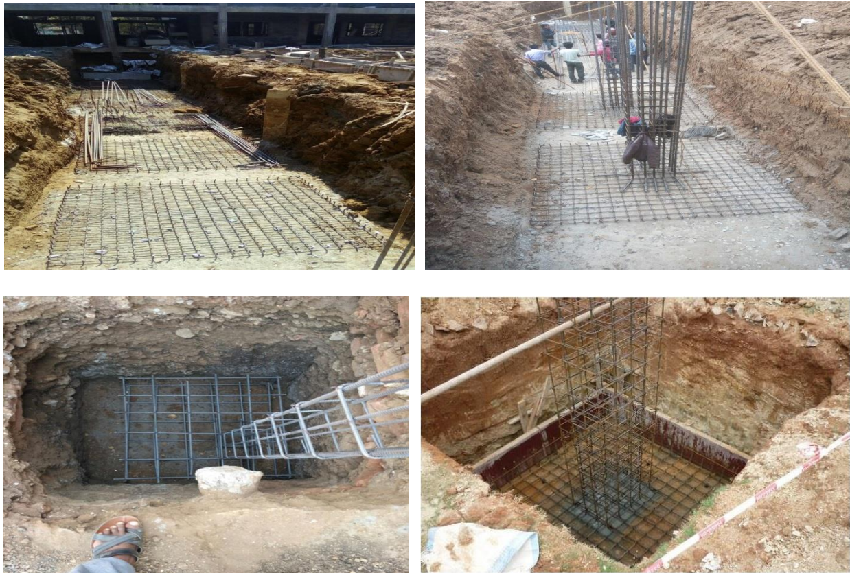
Figure 4 showing the Foundation without PCC
